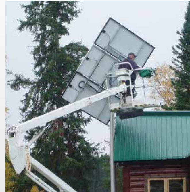
Solar tracker for 3 panels. 0,75 kWp.
