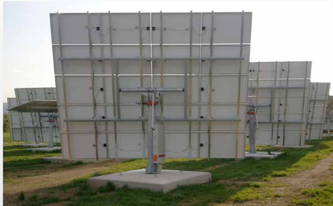
Solar tracker for 15 panels, 441 MWp. Quantity of trackers: 90.
