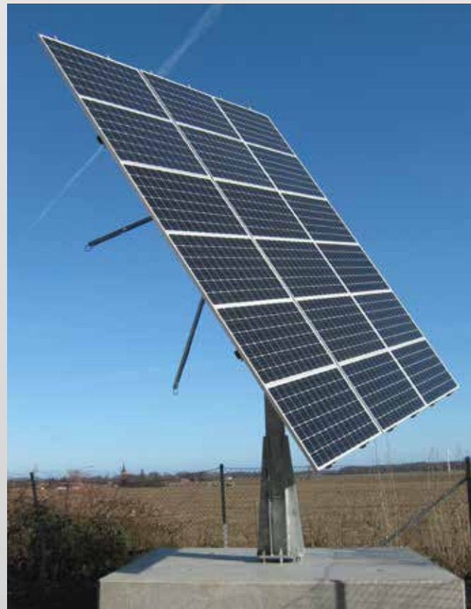
Solar tracker for 18 panels, 16,2 kWp. Quantity of trackers: 3.
