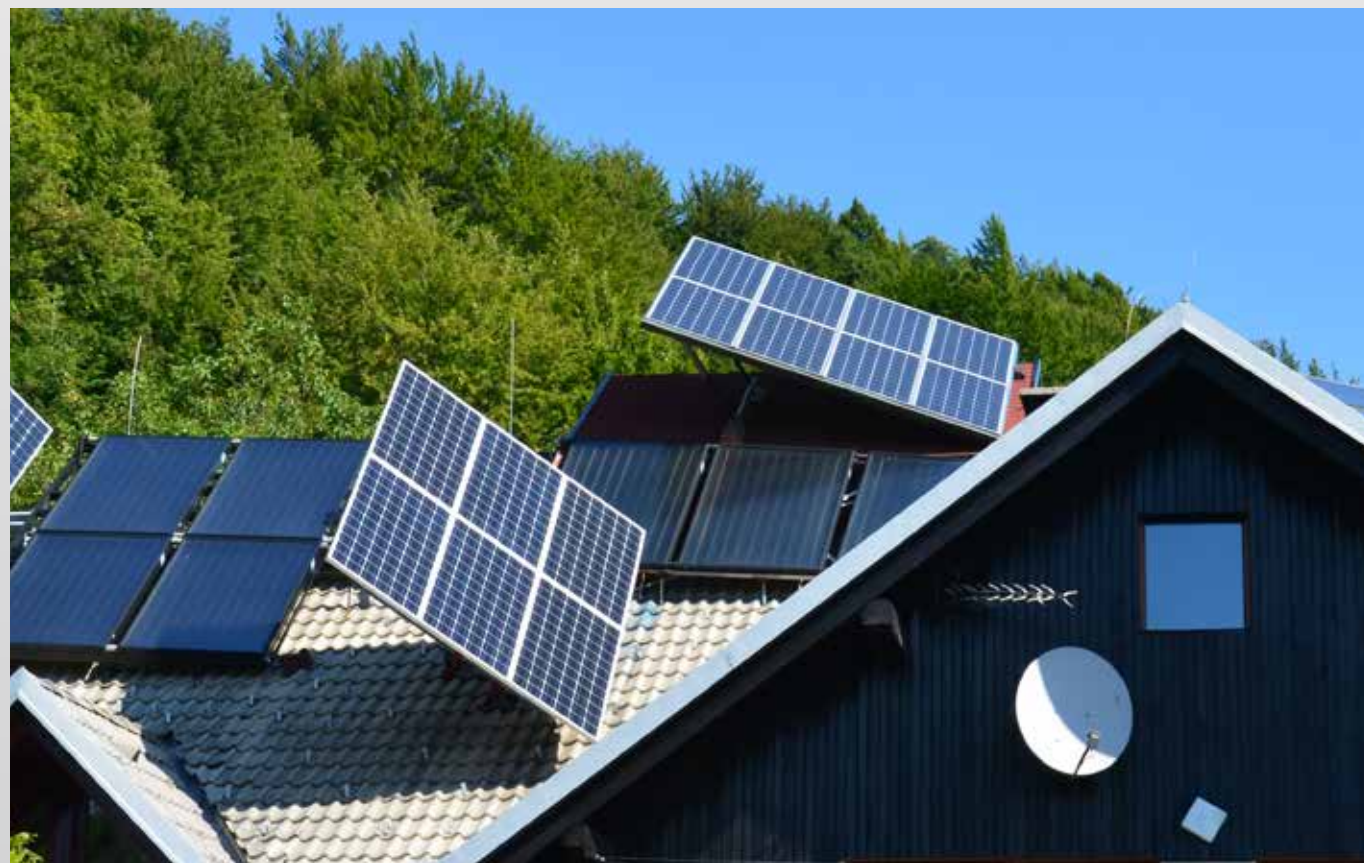
Solar tracker, 4,8 kWp. Quantity of trackers: 3.
