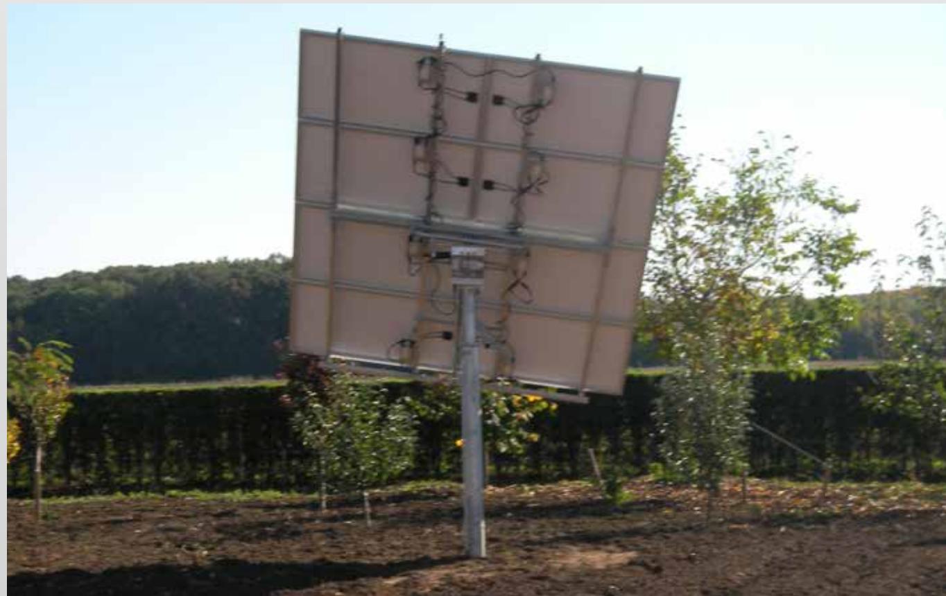
Solar tracker for 15 panels, 3,75 kWp.
