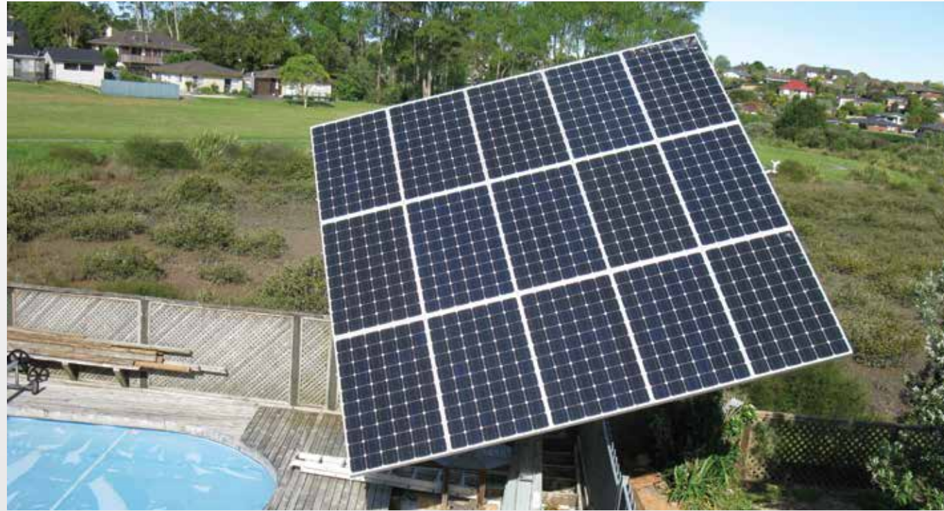
Solar tracker for 15 panels, 3,75 kWp.
